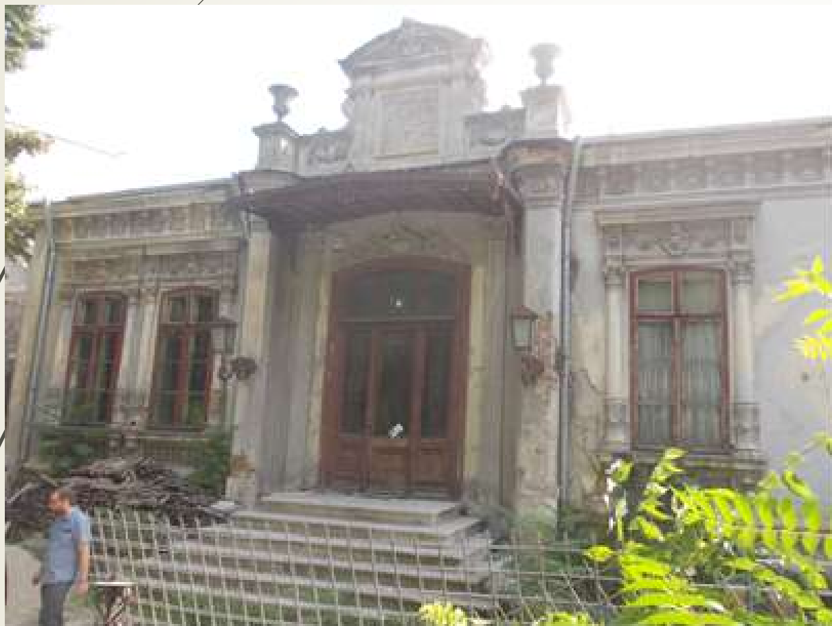
imobil strada dr. R. Calomfirescu nr. 15, sector 3, Bucuresti Subsol partial+Parter+Pod
